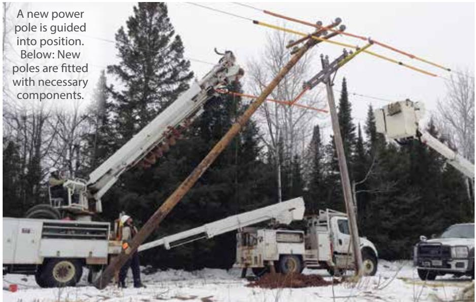
A new power pole is guided into position. Below: New poles are fitted with necessary components.
